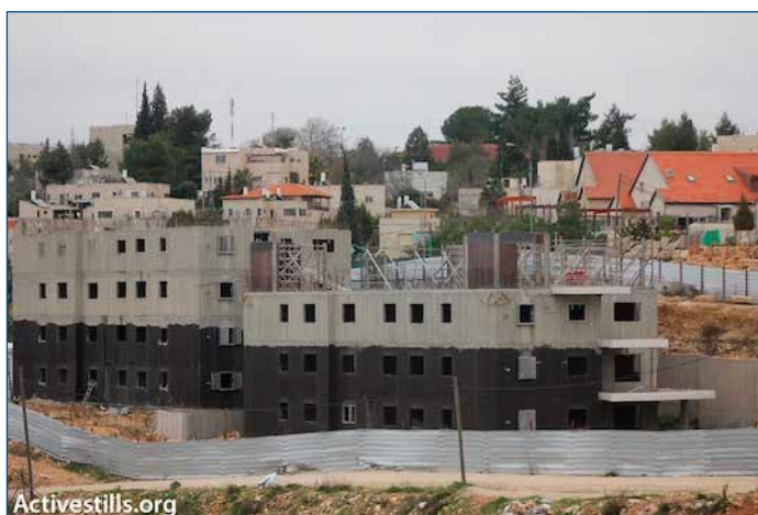
Construction at the settlement of Beit El, February 5, 2013.
